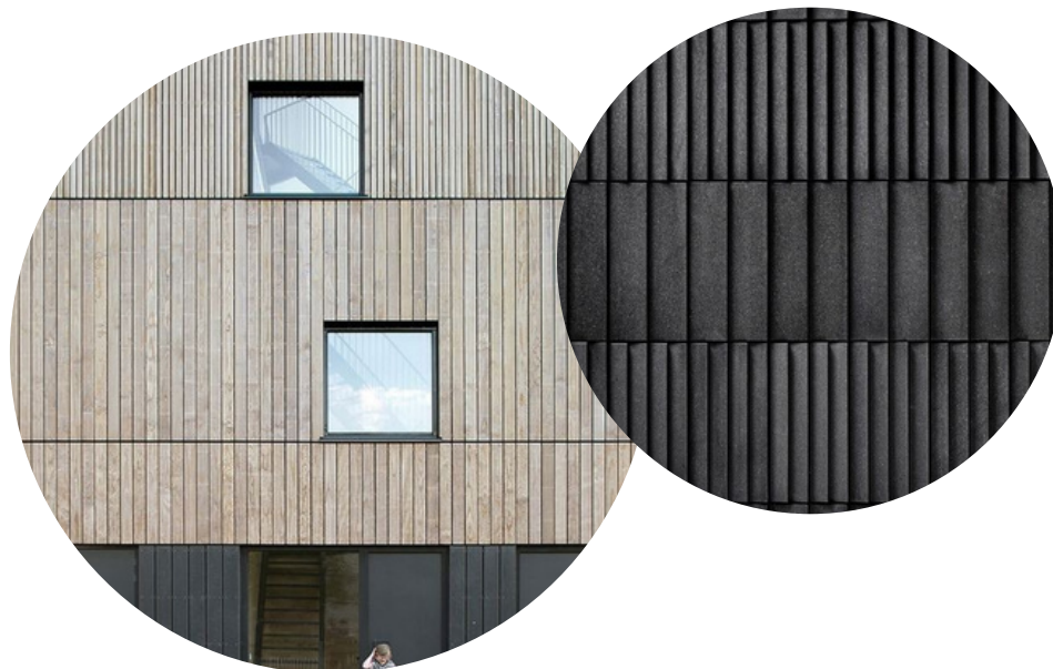
Wood cladding - Planks of different sizes - two tones to distinguish openings in the facade.
